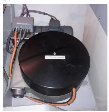
Service on MagnusMaster is minimal with very occasional greasing of the upper mechanism (via external, easily accessible grease nipples) and seal changes in the leisure market being set at 5 years (or equivalent in a commercial application depending on hours operational).
