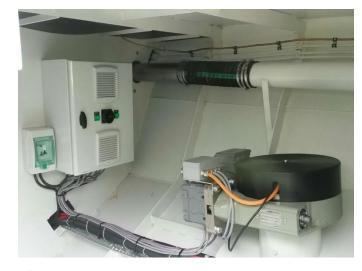
The control cabinet does not have to be in the same location/vicinity as the primary motor drive unit as long as appropriate connecting cable lengths are pre-determined prior to order.
