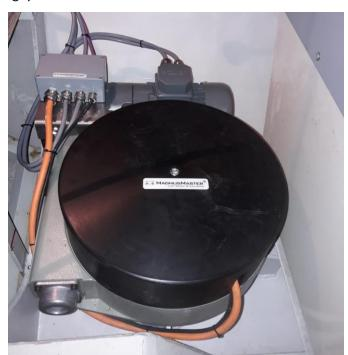
Service on MagnusMaster is minimal with very occasional greasing of the upper mechanism (via external, easily accessible grease nipples) and seal changes in the leisure market being set at 5 years (or equivalent in a commercial application depending on hours operational).
